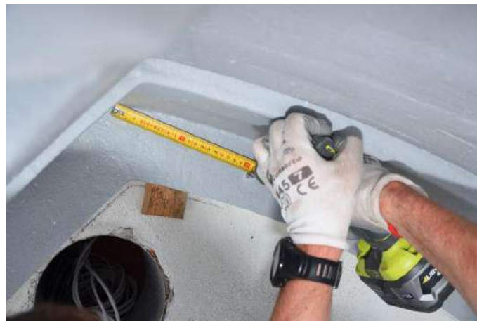
Figure. 12 – drilling of base fixing holes
