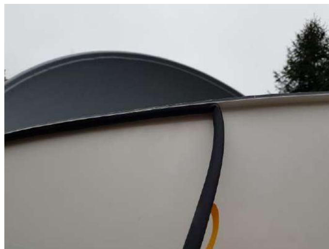
Figure. 67 – mounting the seal on shutter #2
