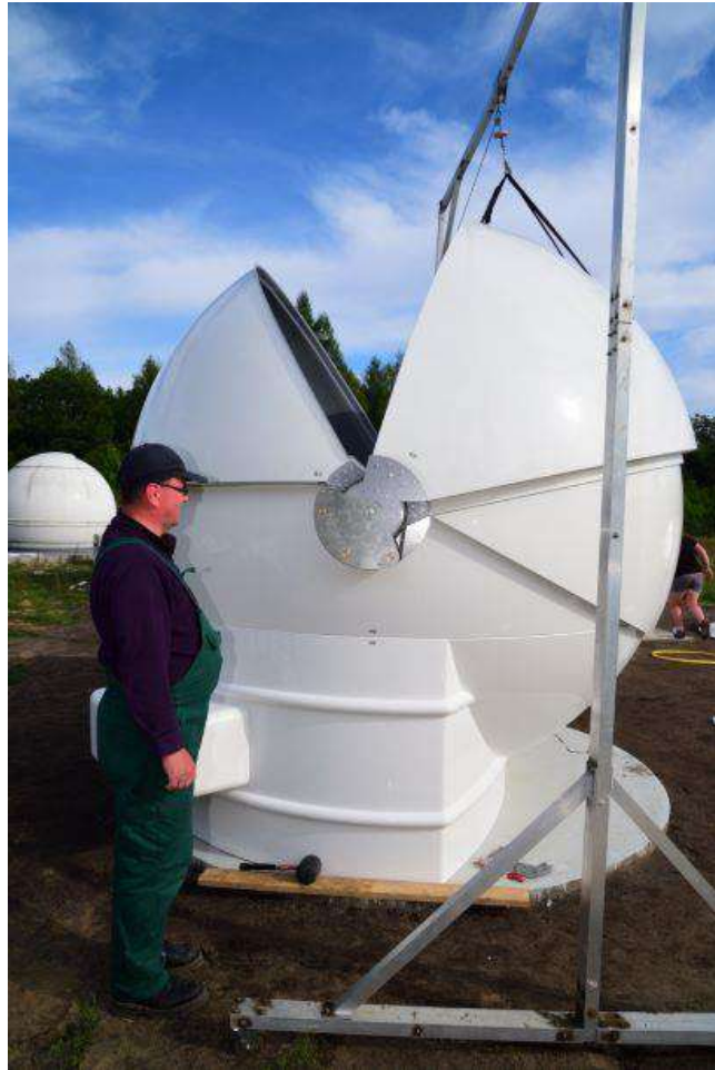
Figure. 54 – mounted shutter No. 3 mounting in its handles
