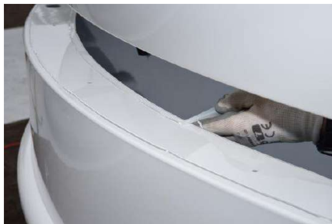
Figure. 21 – sealing of the observatory base elements
