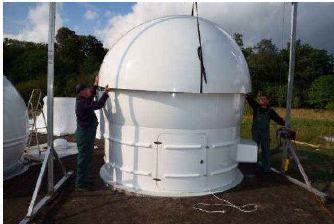
Figure. 39 – Shutter no. 1 placed on the ring of the base.
