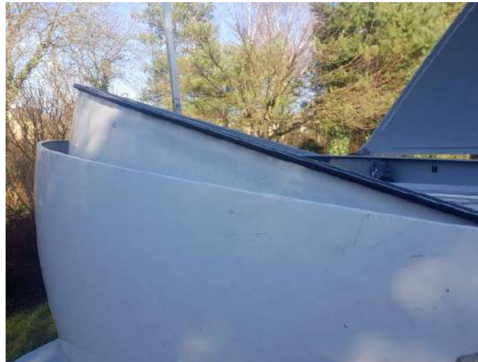
Figure. 66 – Opening of shutter #2 for seal mounting
