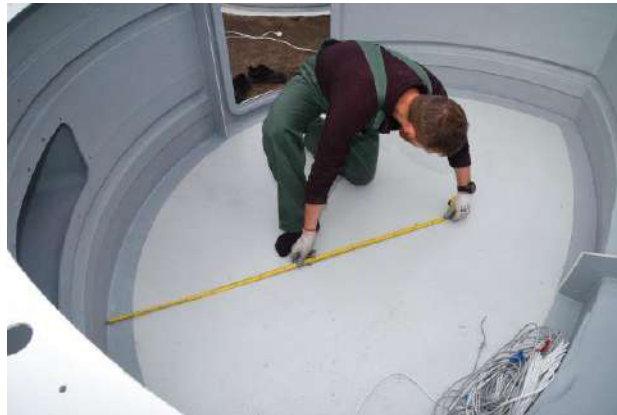
Figure. 8 – positioning of the bases of the observatory
