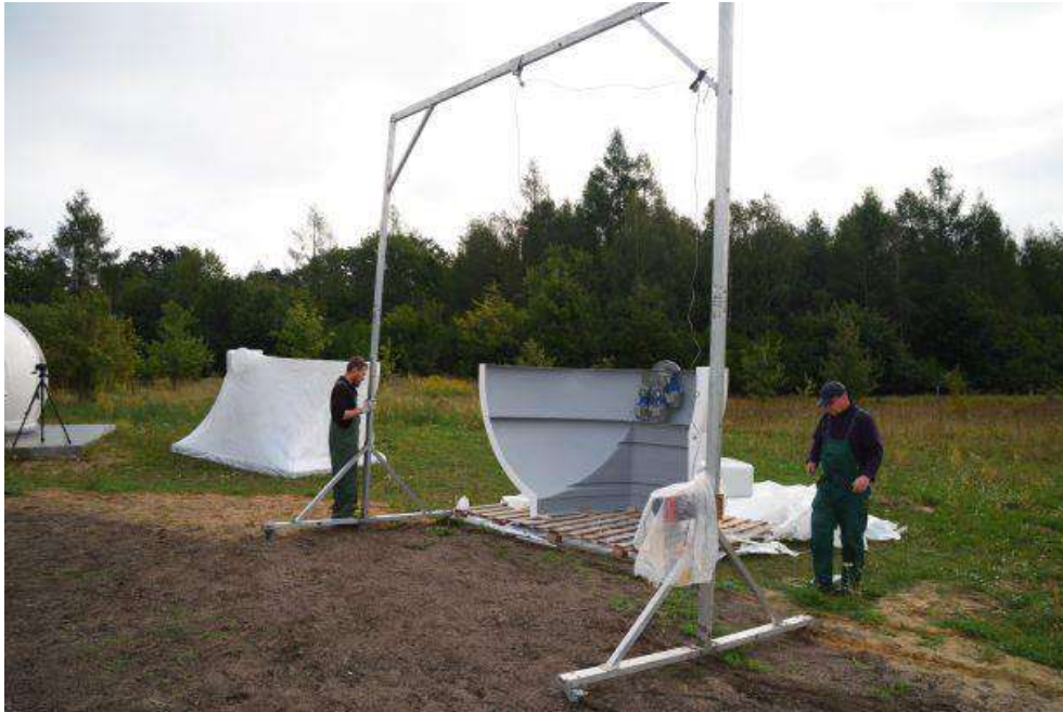
Figure. 4 – electric gantry used for observatory mounting
