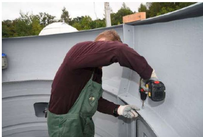
Figure. 25 – Final connection of the upper elements of the observatory base with screws
