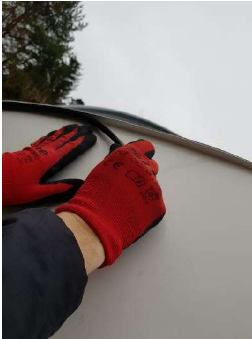
Figure. 68 – mounting the seal on edge of shutter #2
