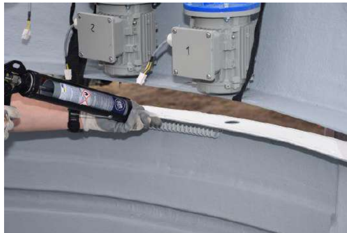
Figure. 20 – sealing of the observatory base elements
