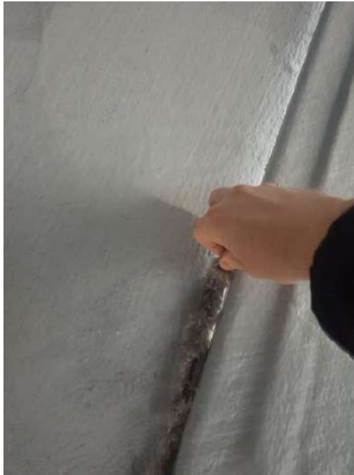
Figure. 70 – Installation of the gasket on cover 3
