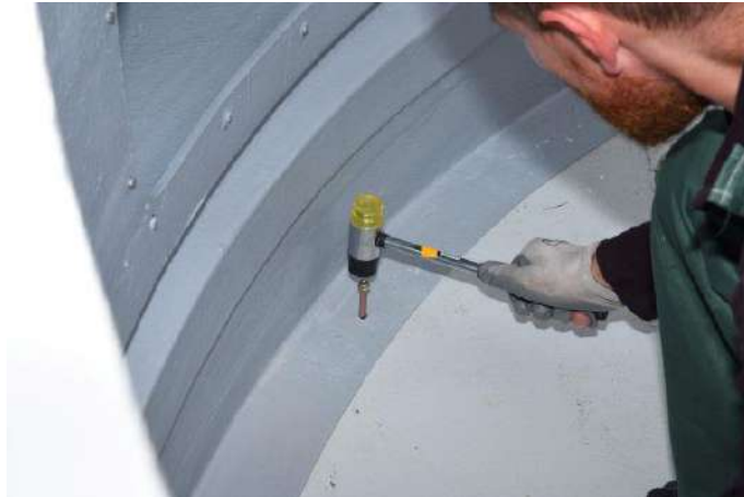
Figure. 17 – mounting the base with anchors
