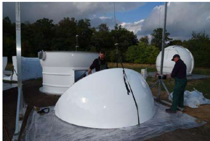
Figure. 37 – Shutter No. 1 – orientation before installation
