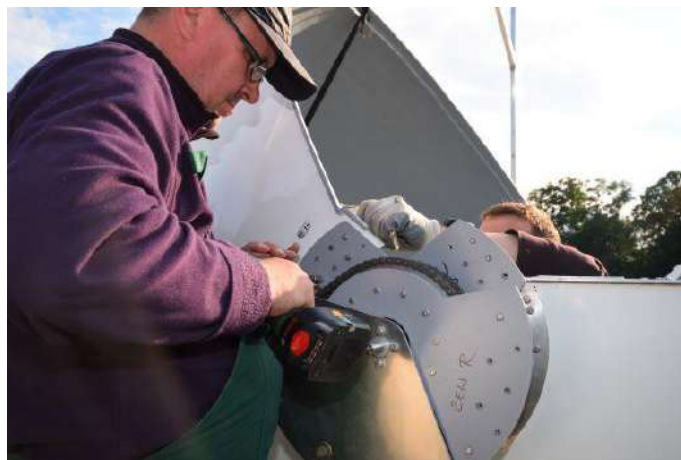
Figure. 42 – screwing the shutter #1 to its mounting handle
