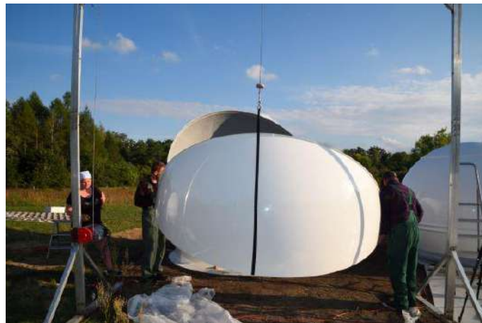
Figure. 47 – shutter No2 transport to top of base
