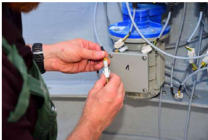
Figure. 33 – connecting the motor power wires on the left side of the observatory base to the controller
