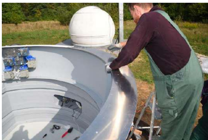
Figure. 29 – Securing the ring with mounting screws
