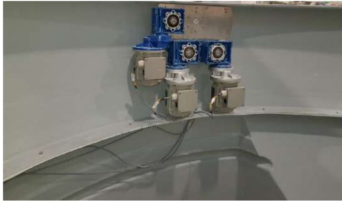
Figure. 32 – power connection wires for the left side of the observatory base
